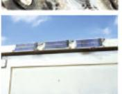
Three of 16 Industrial 12-Volt Solargizers maintaining the backup batteries on a railroad crossing signal.
