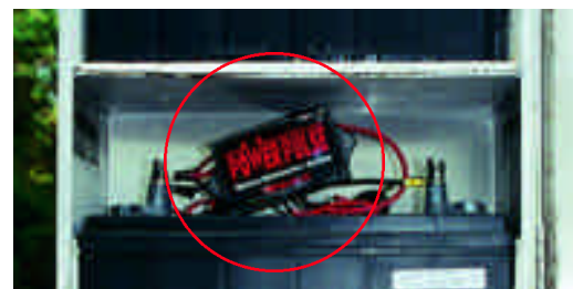
Photos: (Top) Solar-powered school zone flasher with a 12-Volt PowerPulse installed on the battery (bottom).
